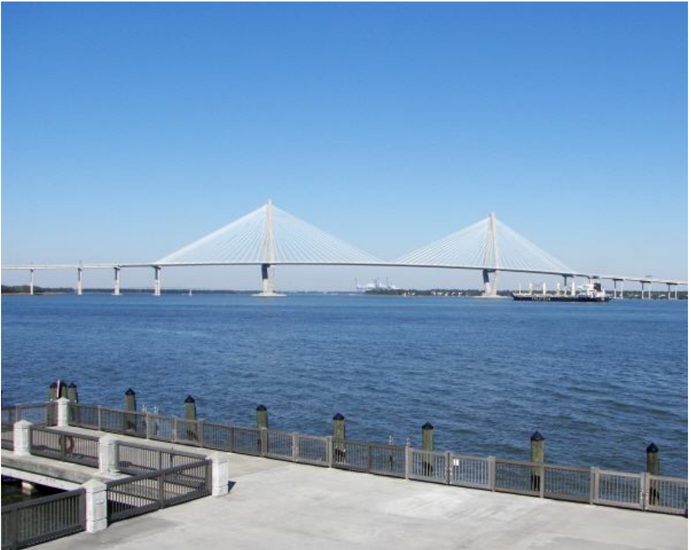
Arthur Ravenel Jr. Bridge across Charleston Harbor
